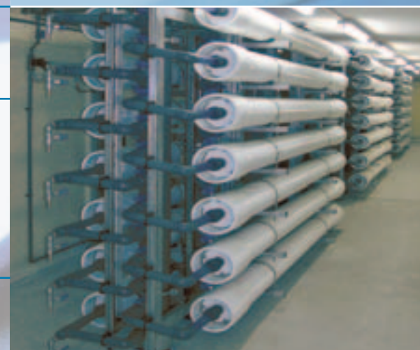
Reverse Osmosis in PVC-U for Municipal membrane systems.
