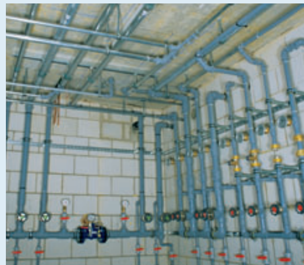
Hot and cold water piping system in INSTAFLEX® PB.
