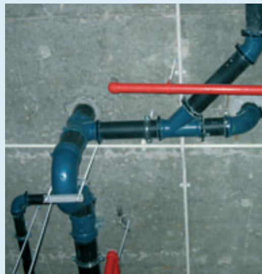
Chemical drain and waste system in FUSEAL® (PVDF/PP).
