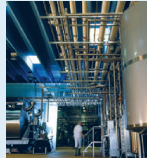
Refrigeration and cooling system in pre-insulated ABS with COOL-FIT™.
