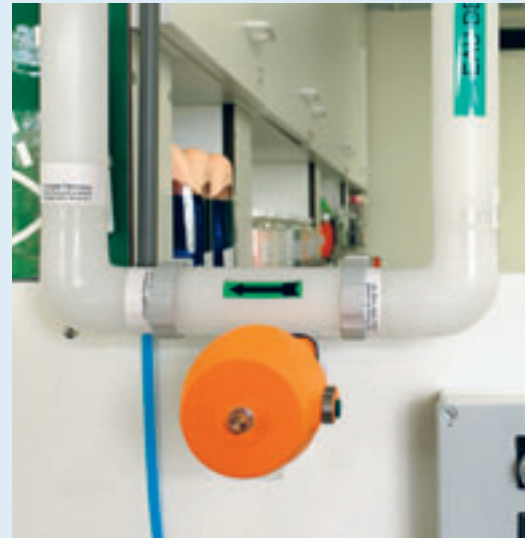
Pharmaceutical water distribution in SYGEF® (PVDF).
