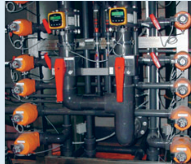
Water treatment in PVC-U, PVC-C, ABS and (β)-PP-H.
