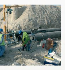
The butt-fusion welding cycle of thermoplastic pipes (PE, PP, PVDF) consists of a certain number of steps. The quality of welding joints depends on the skill of the welder, the suitability of the equipment used and the compliance to the applicable welding standards. The time and pressure values are given by country specific recommendations.
